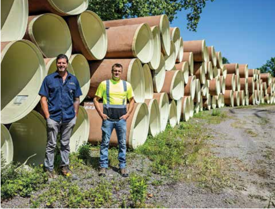
▲ Nick Marra and Chris Berger, general supervisor, at a job site in Cleveland. The piping stacked behind them is part of a 20,000-foot-long sanitary sewer project.
