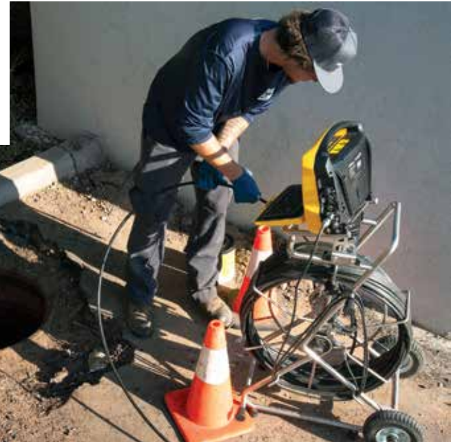
» J.J. Johnson inspects a line using a Vivax-Metrotech camera.
